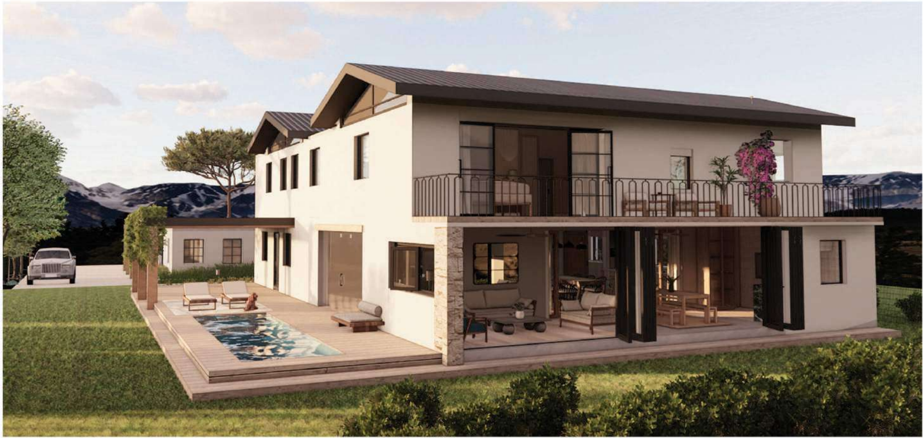
BUILDING VIEW FROM LAGOON
